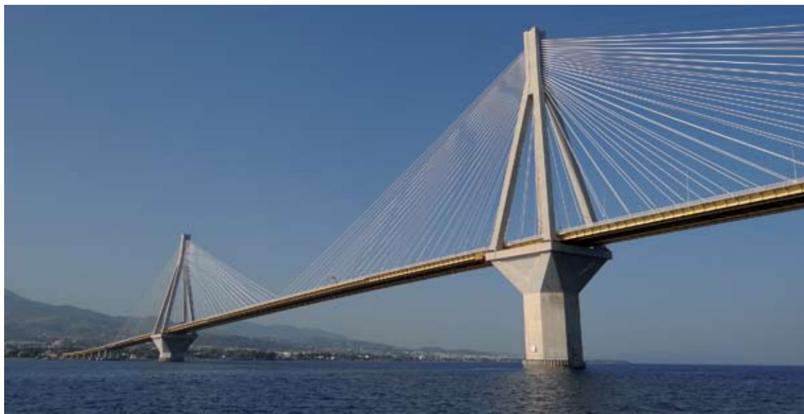
View looking north of part of the Rion-Andirion Bridge which crosses the narrows at the entrance to the Gulf of Corinth.
