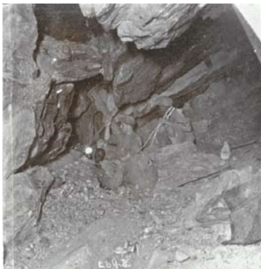
"Charging a pophole C648". The miner is using the steel rod to ram the explosive into the hole while a labourer holds the carbide lamp for light. Note the fuse wire wrapped around one individual's neck!
