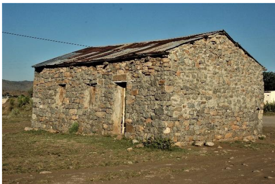
A historical building known as “Merensky’s Office” at Driekop is constructed of dressed blocks of anorthosite
