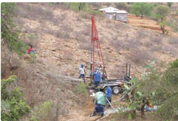
Geotechnical drilling @ km 2.9 bridge sites of Road D4166 at Ga-Riba in Sekhukhune District, Limpopo Province.
