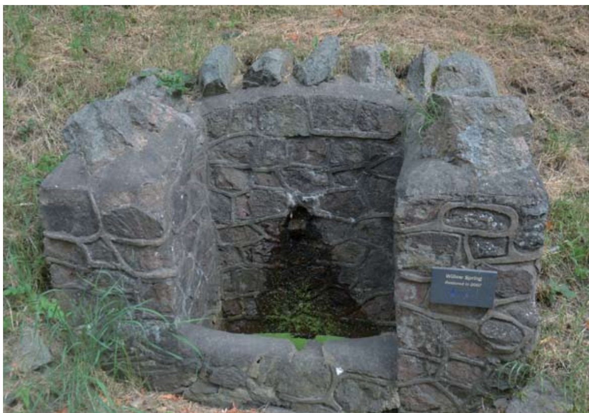
Many of the original springs and wells in the Malvern Hills have been refurbished
