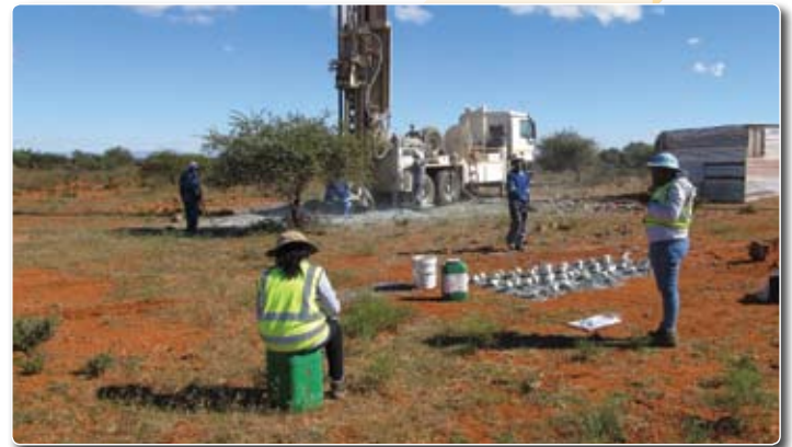
Dolomite stability investigation Skeyfontein located within the jurisdiction of Tsantabane Local Municipality.
