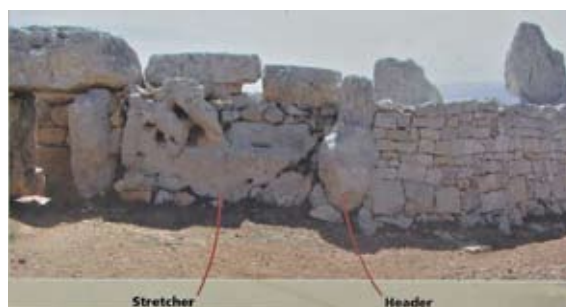
Information board showing usage of “stretchers” and “headers”.
